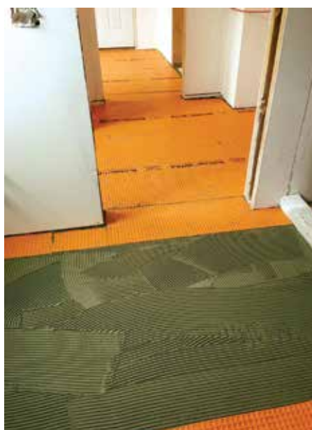
Advantage Schluter Ditra membrane prep
