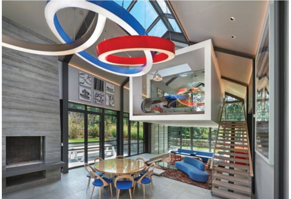
The suspended white square you see is a floating bedroom loft, built using skim coated drywall over a steel frame, and cantilevered off the glass curtain wall.
