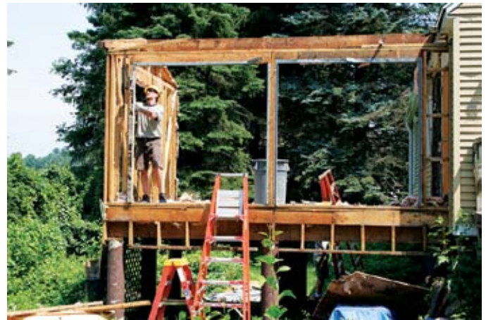
A New England deconstruction in process. Deconstruction saves a large portion of materials from disposal and makes them available for reuse.
