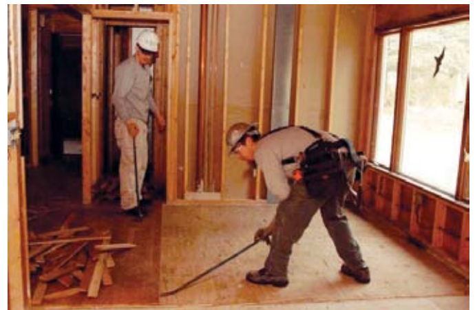
Crews salvaging hardwood floors using a de-nailing process, allowing for reuse.
